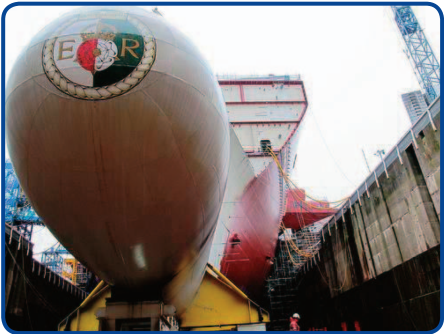
An unusual view of the new aircraft carrier, HMS Queen Elizabeth, in build, dated December 2012
